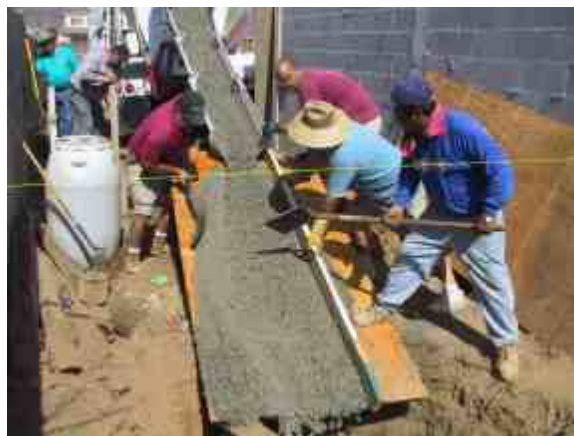
VCC Dublin pouring cement at Pastor Daniel’s church
