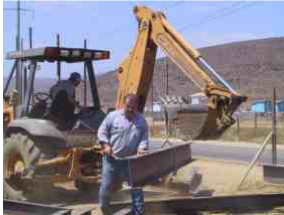
Preparing the beams for Pastor Daniel's church
